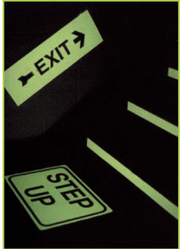
Photoluminescent signage provides positive guidance in “lights out” conditions.
